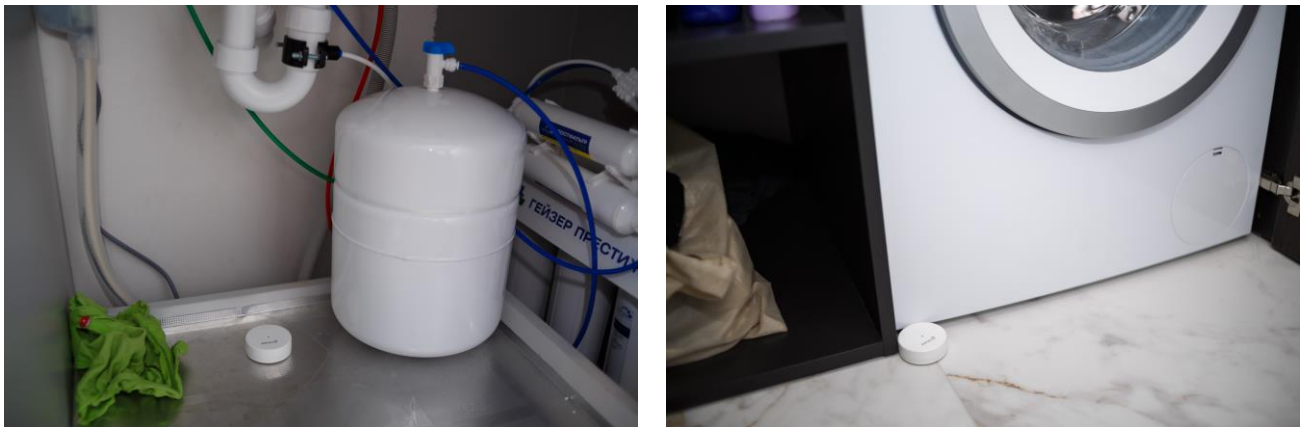
Figure 4 – Examples of Installation of the Leak Sensor
